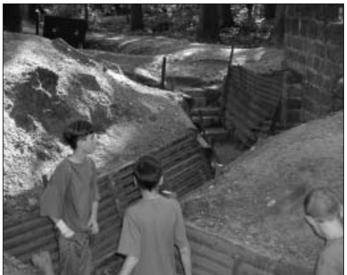
Young men, once more, man the trenches in Ypres
